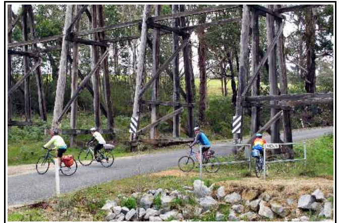
Cyclists under the timber bridge at Wairewa
