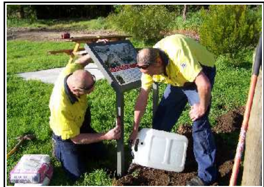
Grant and Jeff installing the boards at the car park.
